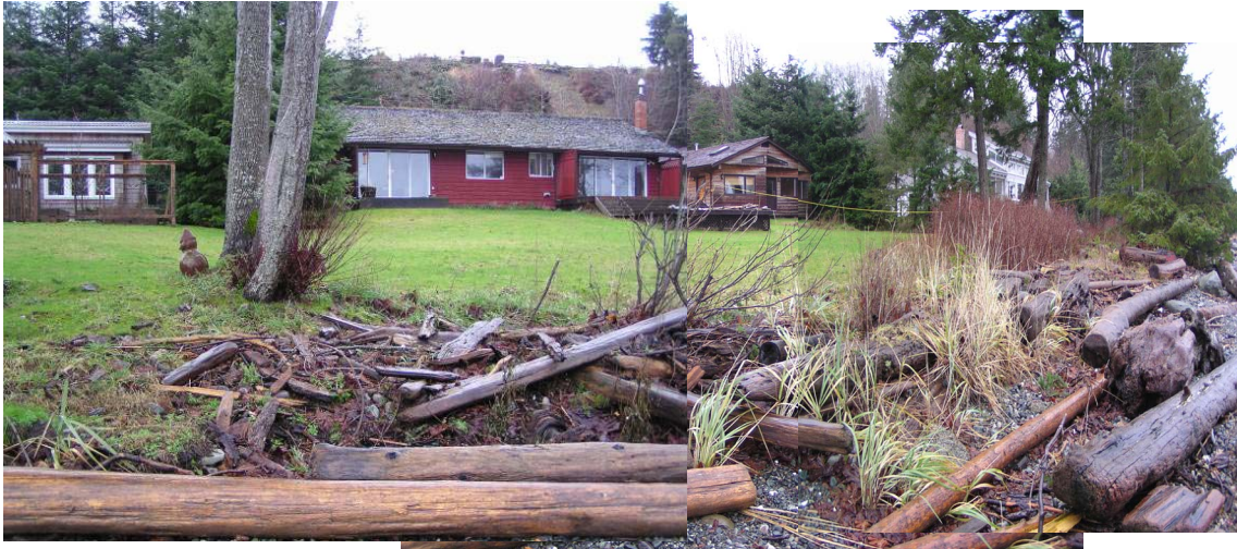
Figure 2. View of the Duncan Property from the foreshore. Coho Drive is between the house and the coastal bluff in the background
