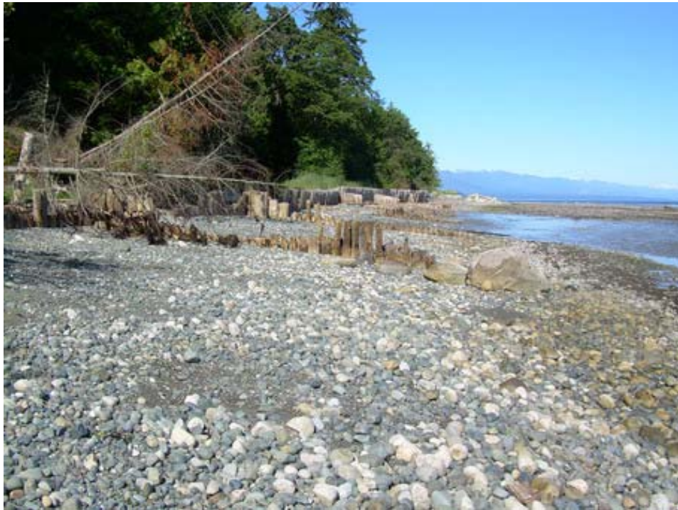
Figure 4. An photo of the beach at Milner Gardens looking alongshore to the northwest. a wooden seawall and groins are visible to the left. The cobble veneer over the beach face is also evident.
