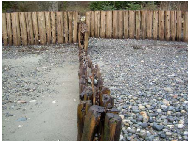
Figure 13. Photo of build-up on right side of groin (west side) indicating right to left sediment transport (to the east) was occurring at the time the photo was taken (March 2007).
