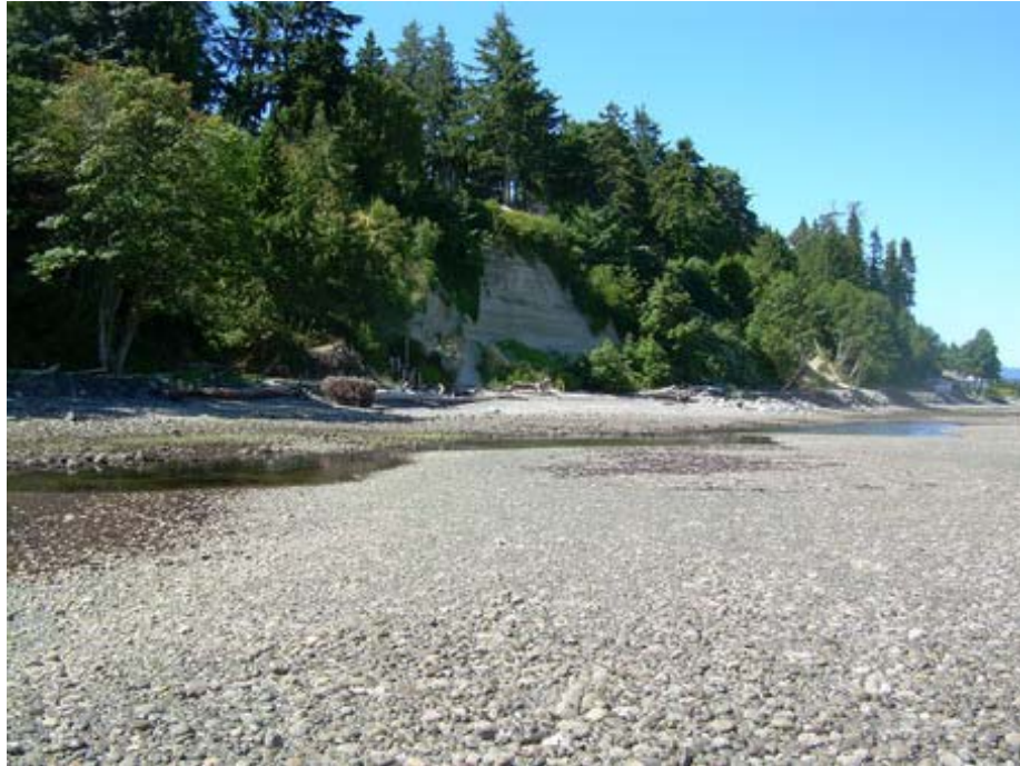
Figure 6. Photo of cliffs to the west of the Mewburn property. Rip-rap placed in the supratidal and intertidal below some of the properties (right portion of photo) to stabilize the cliff toe.
