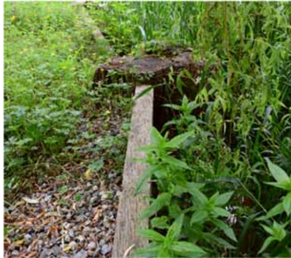
Figure 1: Untreated wood and tree stumps used to stabilize a stream bank
