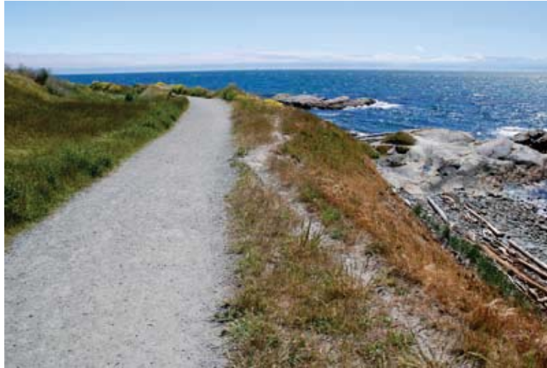
Dogs walking along the edge of this coastal bluff ecosystem in Macaulay Park have created a worn trail, causing excessive erosion and opening the area to invasion by alien species. Photo: Dave Polster
