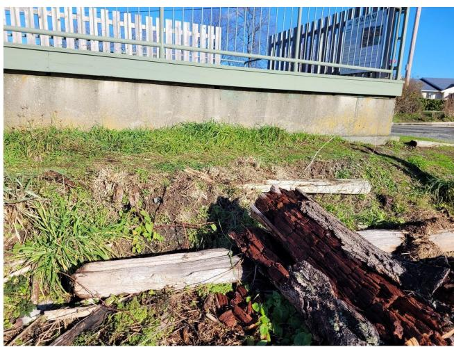
Figure 15 - Seaward side of bird viewing platform with eroding bank below.
