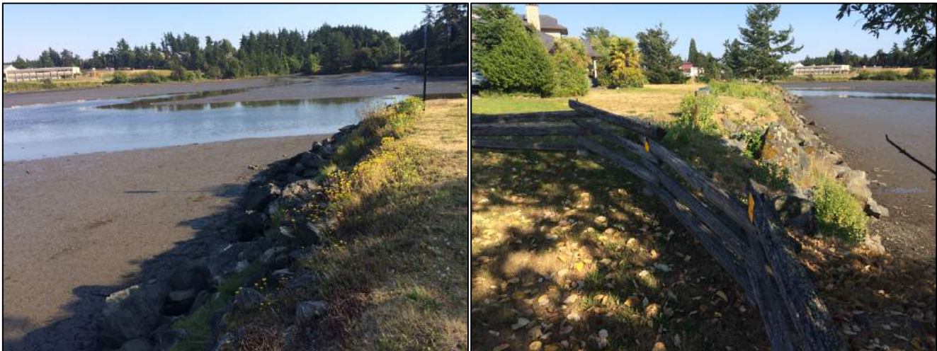
VR11 – Seabird Pl riprap shoreline adjacent to portage Inlet (left) and ROW (right).
