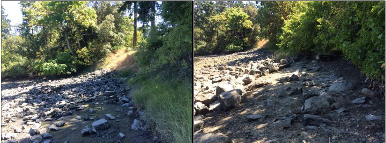
V01 – Emergent shoreline vegetation present under native overhang, but missing under ivy and daphne vergrowth.
