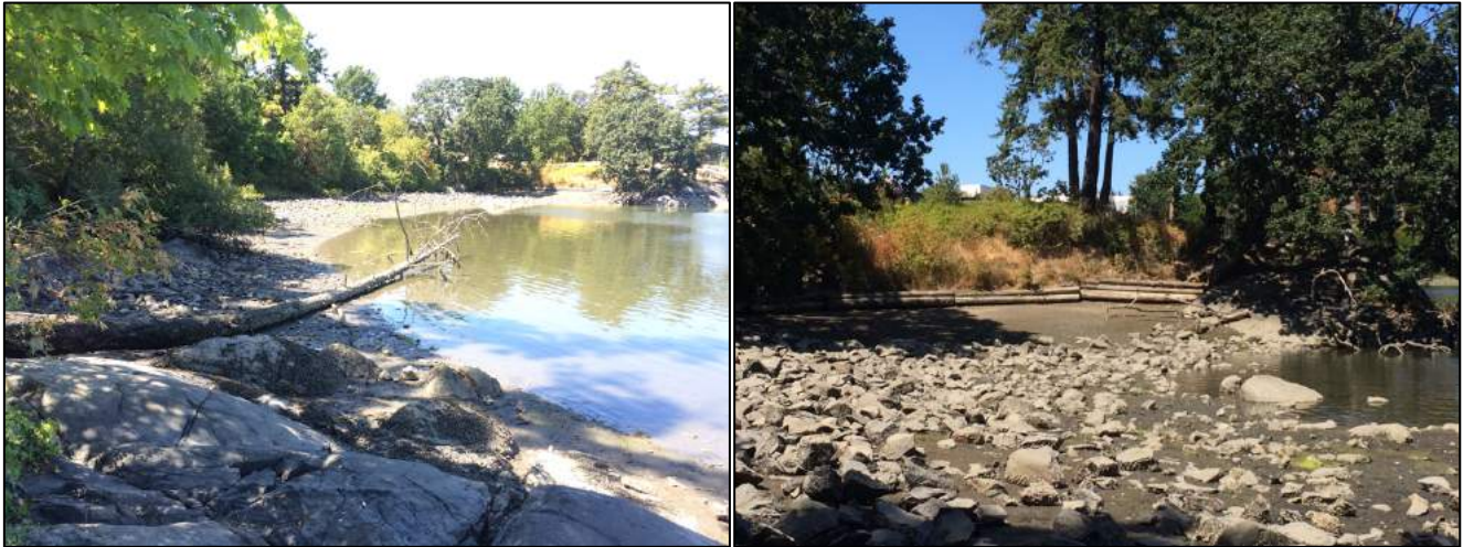
V01 – Banfield Park western cove. Riprap covers most of beach, but not slopes. Previous bioengineering on some slopes.
