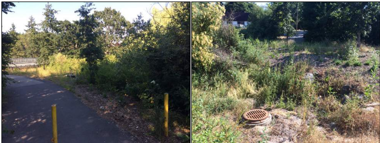
S08- Colquitz Park @ Colquitz Ave ROW & pedestrian/cycling access (left) & raised stormwater drain and weedy bed (right).
