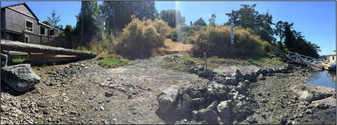
V02 – Previously restored shoreline project involved bulkhead removal, beach creation and shoreline planting.
