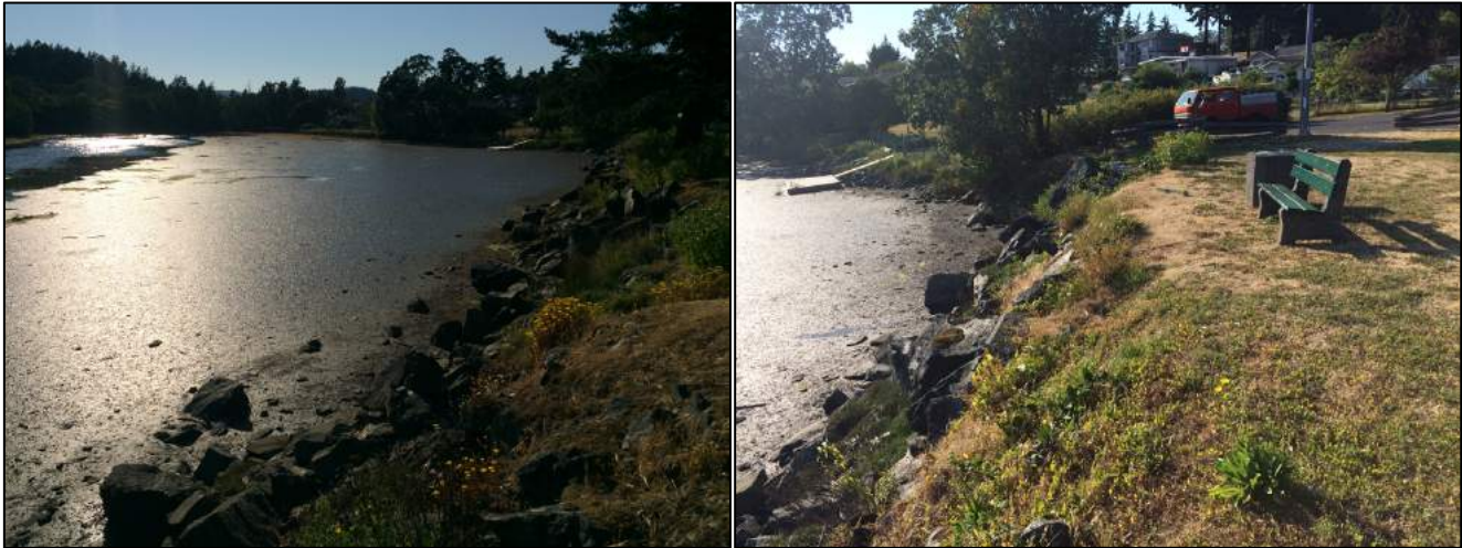
VR11 – Seabird Pl riprap shoreline adjacent to Craigflower Creek estuary mudflats (left) and ROW (right).
