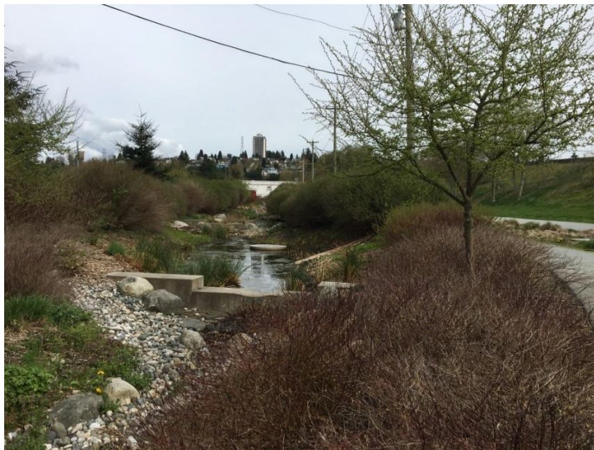
Figure 12. Example of a bioswale used to filter runoff, New Brighton Park, Vancouver BC (Coastal Geologic Services, 2018).
