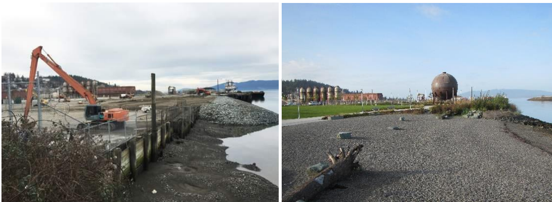
Figure 15. Armour removal and retreat project at Waypoint Park in Bellingham, Washington, (US), designed to accommodate significant sea level rise. Left: before removal. Right: current active beach (Coastal Geologic Services Inc.).
