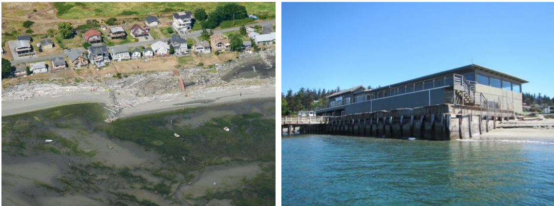
Figure 8. Examples of groynes: rock structure (left), overwater building (right). Both structures trap littoral sediment transport and reduce the volume of sediment that is able to bypass the structure (Coastal Geologic Services, Inc.).
